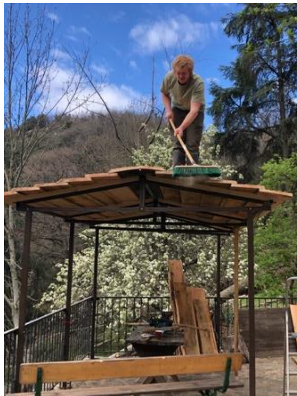
Max working on the pergola roof
