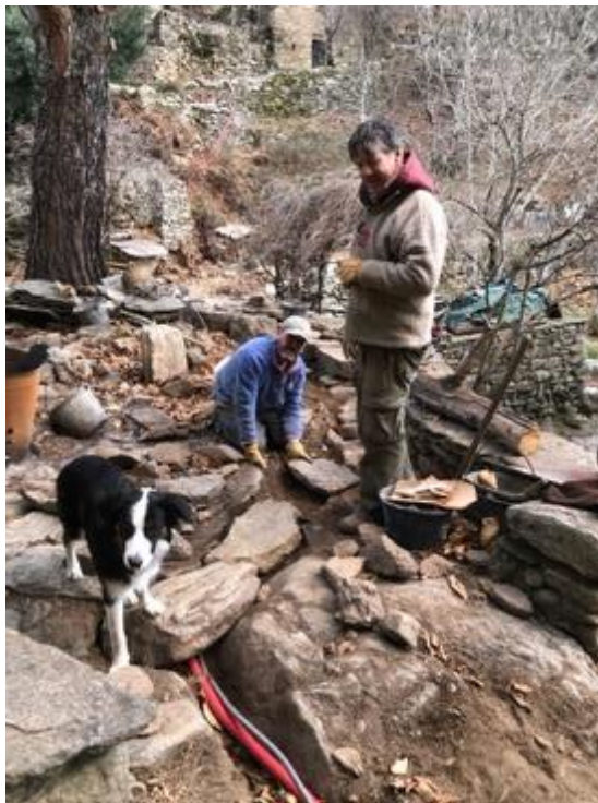
Brian, Ken and Seamus laying the Optic Fiber
